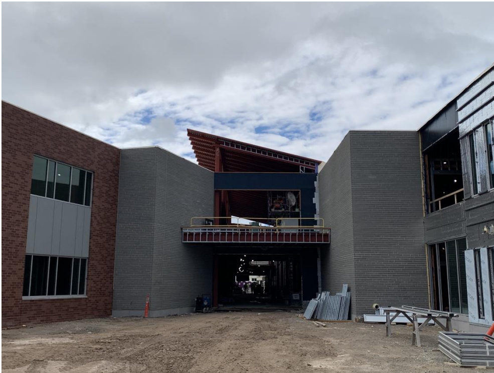
7. Area 4 East – Board insulation, sub girt system, and composite metal panel installation in progress.
