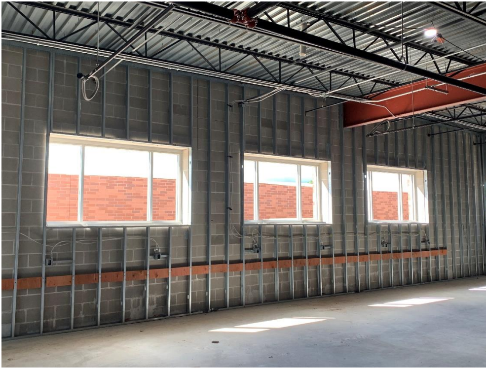
31. Area 3 Second Floor – Gradewing entry feature blocking and framing installation in progress.
