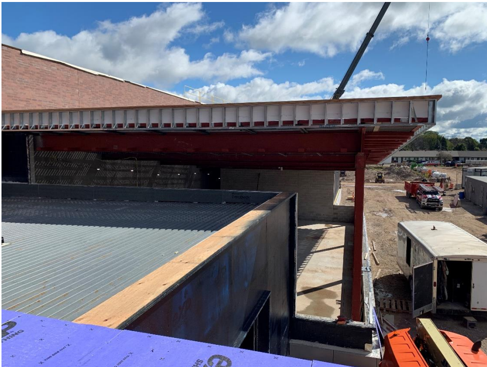
29. Area 1A/2B – Roof decking installed. Exterior cold form framing installation in progress.
