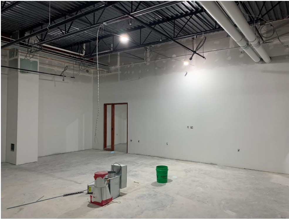
15. Area 5 – Gyp board installation in stairwell corridor in progress.
