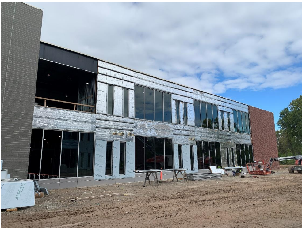
7. Area 4 East – Board insulation, sub girt system, and composite metal panel installation in progress.
