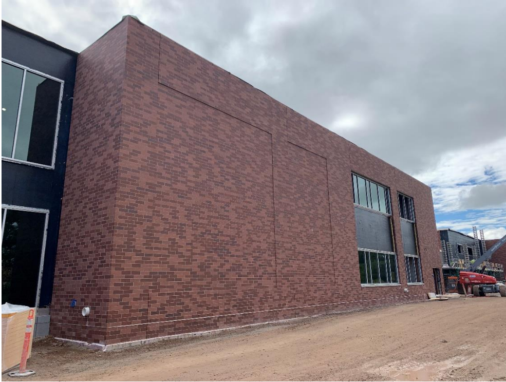
11. Area 3 West – Cast stone panels installed. Exterior brick veneer installation in progress.
