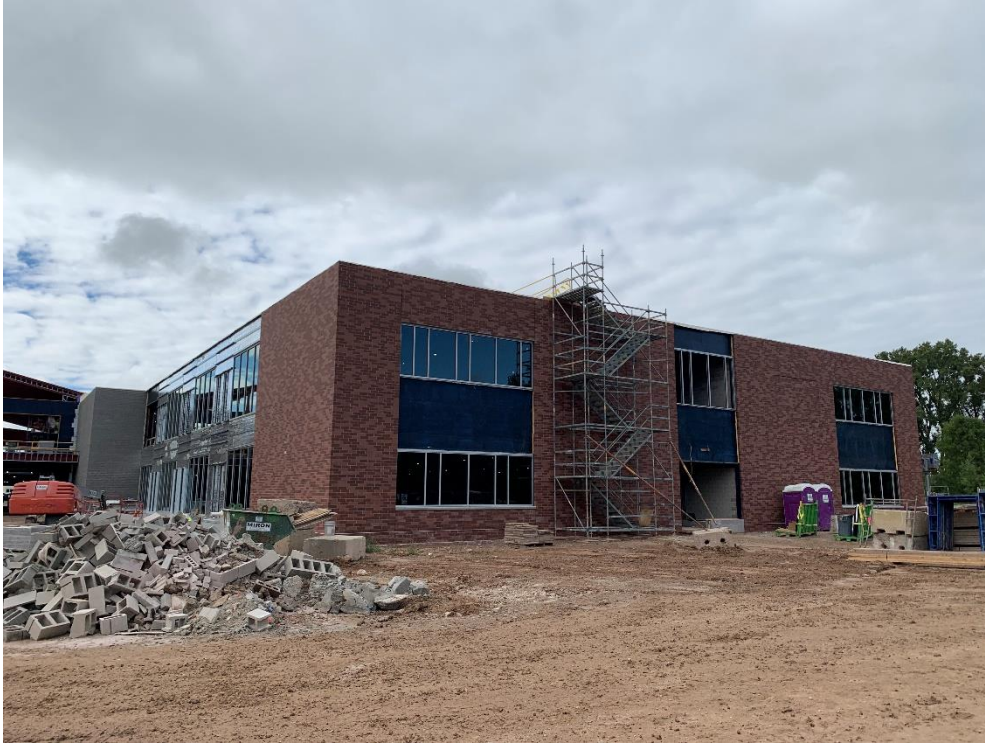
9. Area 4 West – Board insulation, sub girt system, and storefront glazing installation in progress.
