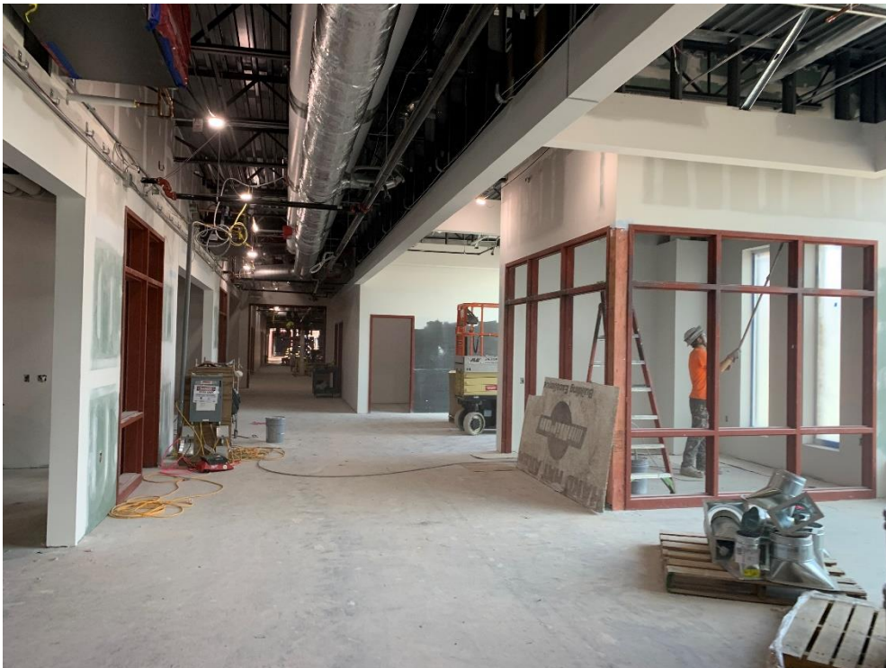
13. Area 6 – gyp board taping, mudding, and priming in progress.
