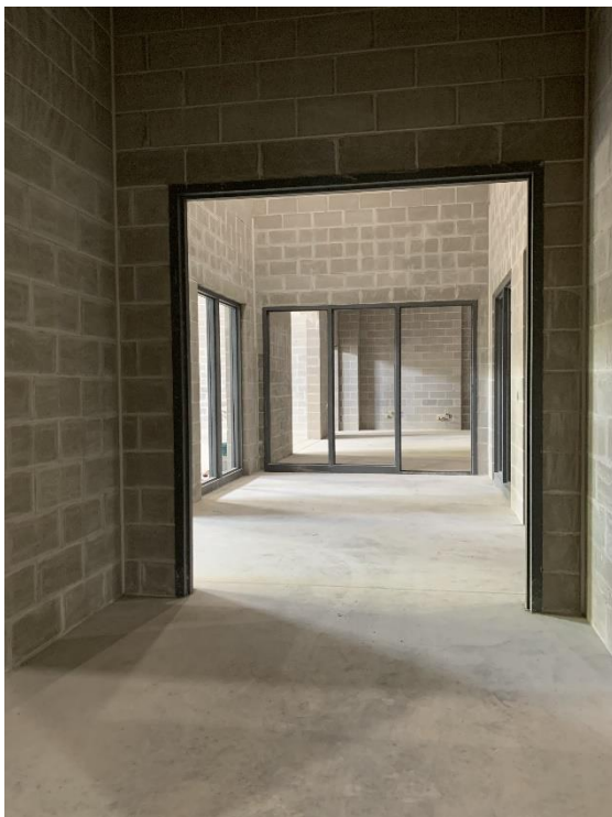
35. Area 3 – Interior cmu walls and hollow metal frames installed in tech ed area.
