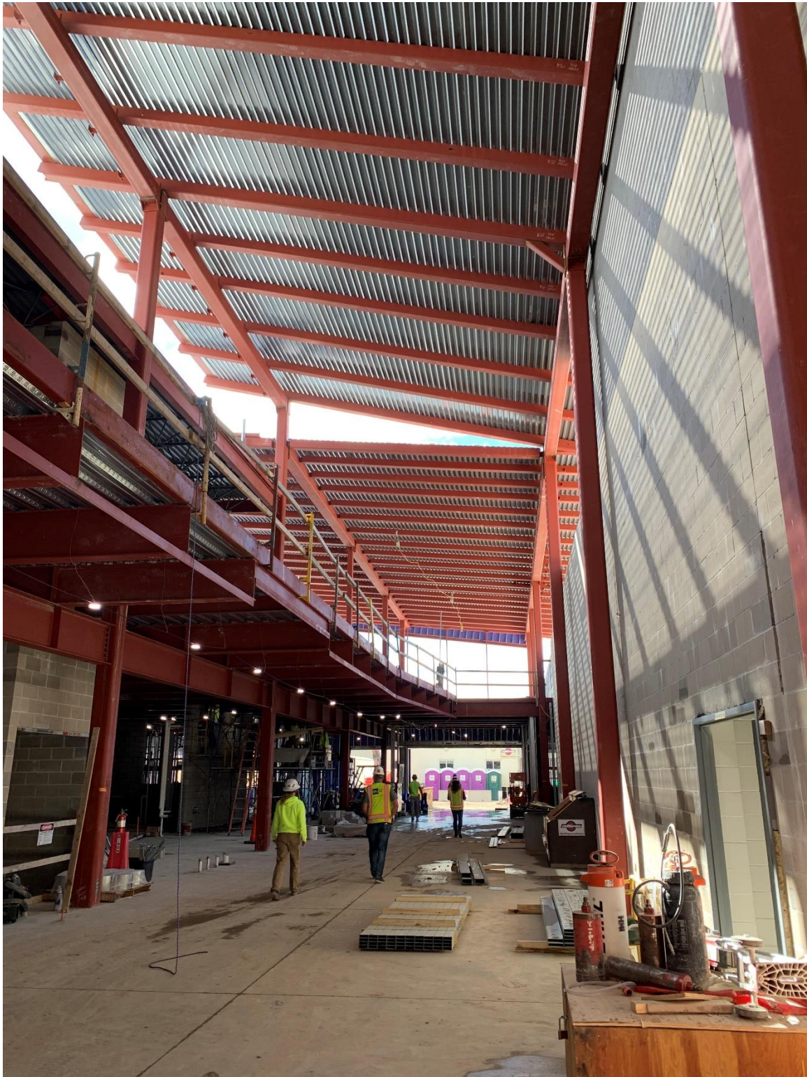
36. Area 1A – Acoustic roof decking installed in center spine.
