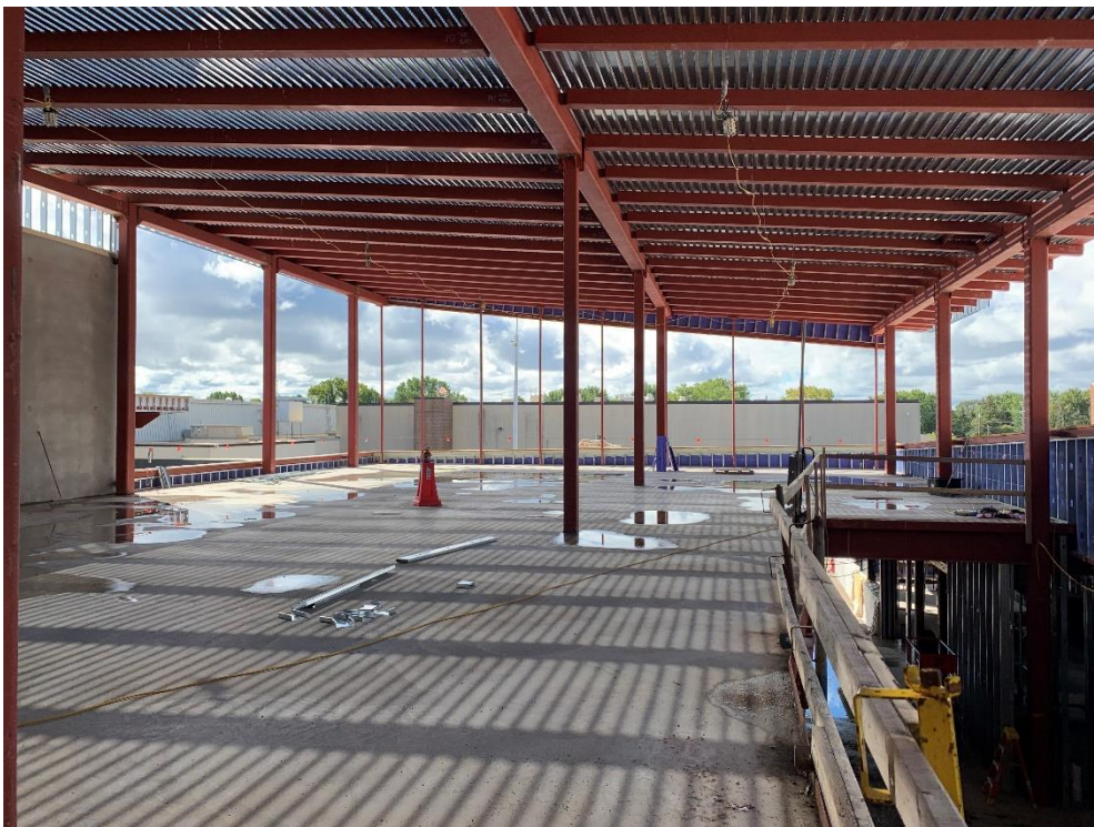
27. Area 1A Second Floor – Acoustic roof decking installed.
