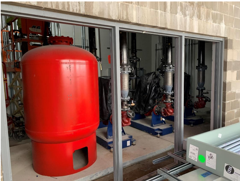
21. Area 1B First Floor – Geothermal pump room equipment installation in progress.
