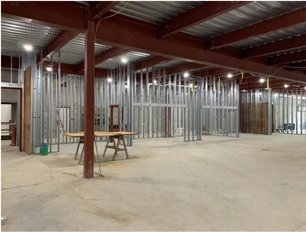
23. Area 4 First Floor – Interior metal stud framing, blocking, and in wall conduit installation in progress.
