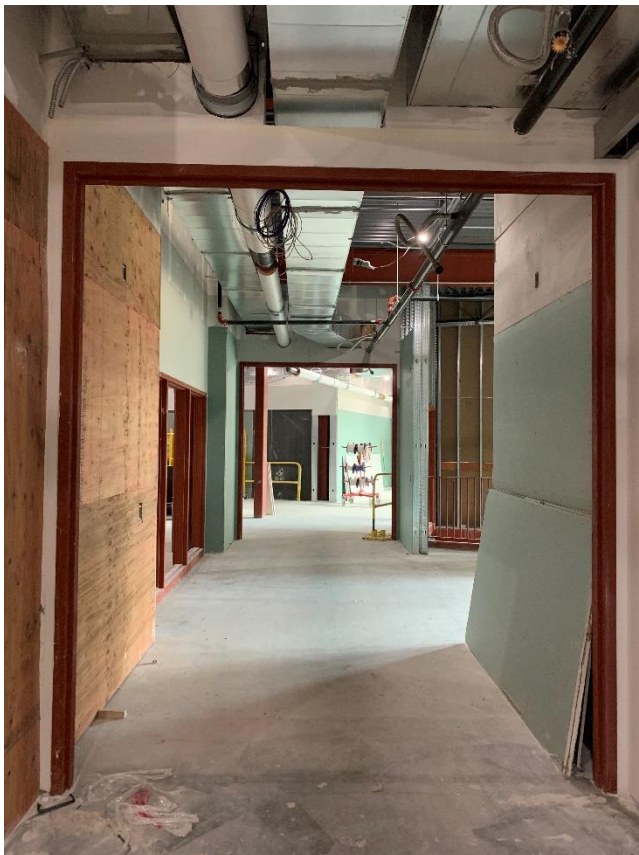
15. Area 5 – Gyp board installation in stairwell corridor in progress.
