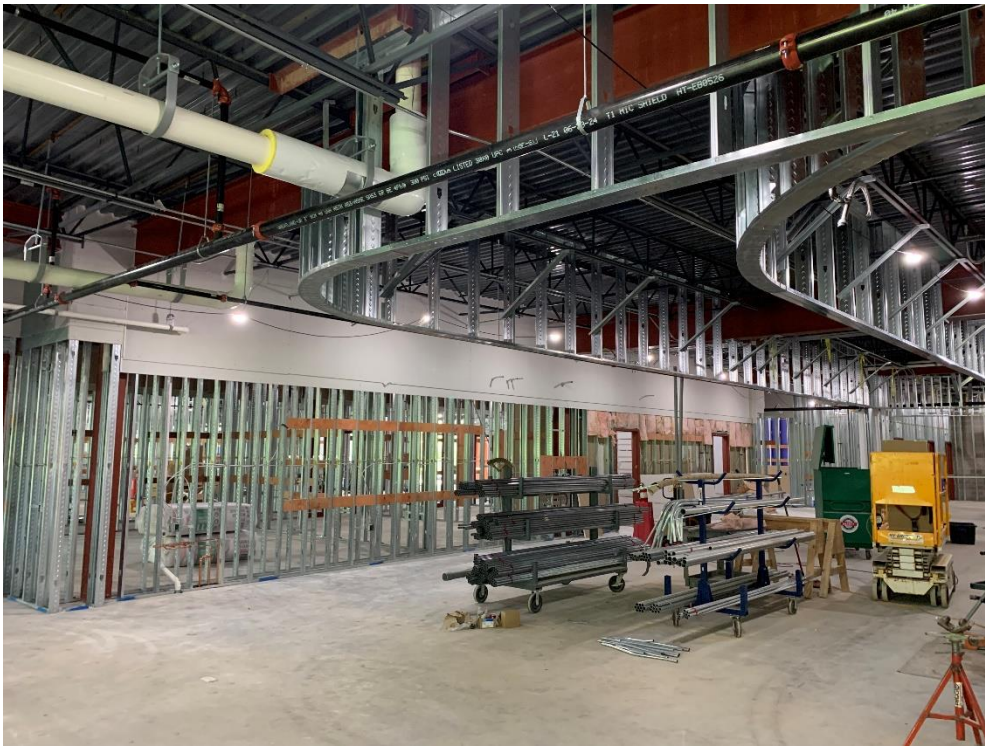
27. Area 1A Second Floor – Acoustic roof decking installed.
