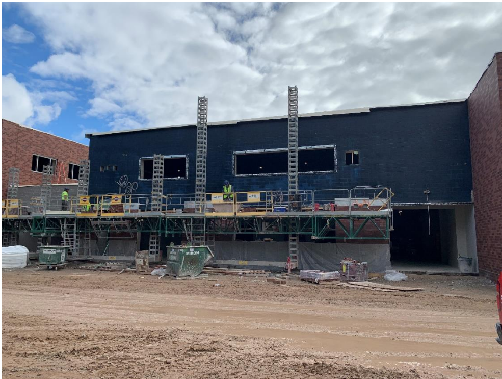
11. Area 3 West – Cast stone panels installed. Exterior brick veneer installation in progress.
