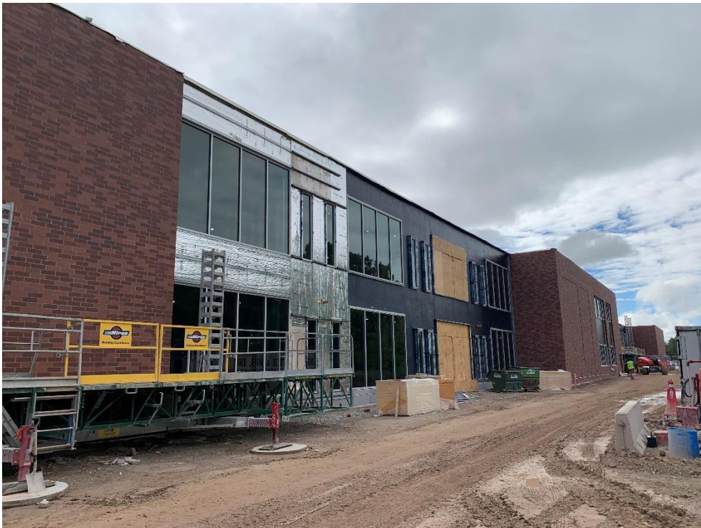
9. Area 4 West – Board insulation, sub girt system, and storefront glazing installation in progress.
