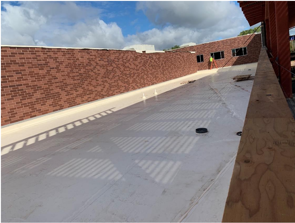
29. Area 1A/2B – Roof decking installed. Exterior cold form framing installation in progress.
