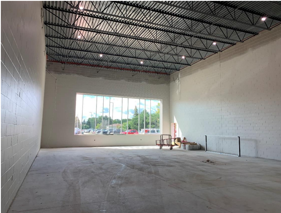
35. Area 3 – Interior cmu walls and hollow metal frames installed in tech ed area.
